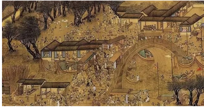
Figure 28 Bamboo Lock Bridge in Song Dynasty Source: The National Palace Museum
